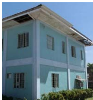
Fig.8-12. Slightly damaged buildings (roof and windows) in Medellin, Cebu.
