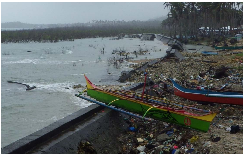
Fig.5-32. Damage to the Hernani seawall. Crest height 3 m above Mean Sea Level.
