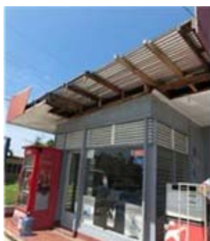
Fig.8-12. Slightly damaged buildings (roof and windows) in Medellin, Cebu.
