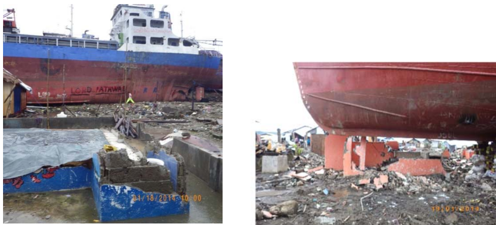
Fig.5-14. Flattening of houses by a drifting ship in coastal Tacloban.
