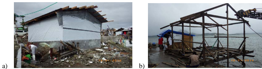
Fig.5-11. a) A house rebuilt with corrugated galvanized iron sheet and wooden studs, b) A house being rebuilt with debris.
