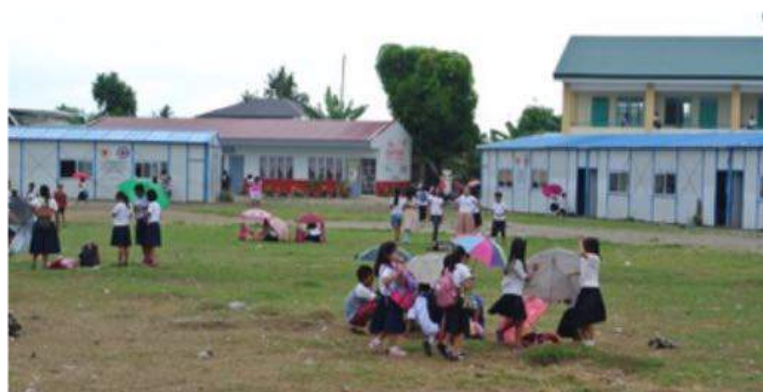
Figure 4.2 Temporary learning spaces and newly built classrooms and reconstructed buildings in the school yard (San Jose, ES, January 2016)
