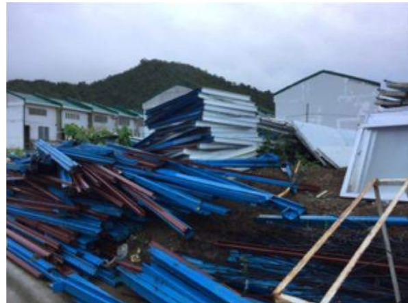
Figure 4.4 Demolished TLS materials in Ridgeview (January 2016)
