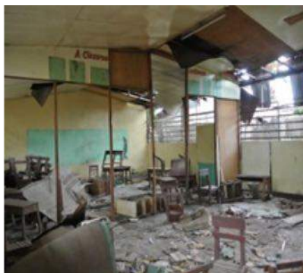
Figure 4.1 Damaged classroom (San Jose ES, July 2015)
