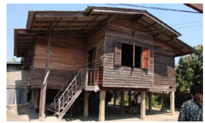
example of traditional housing repaired in Sai Kao subdistrict
