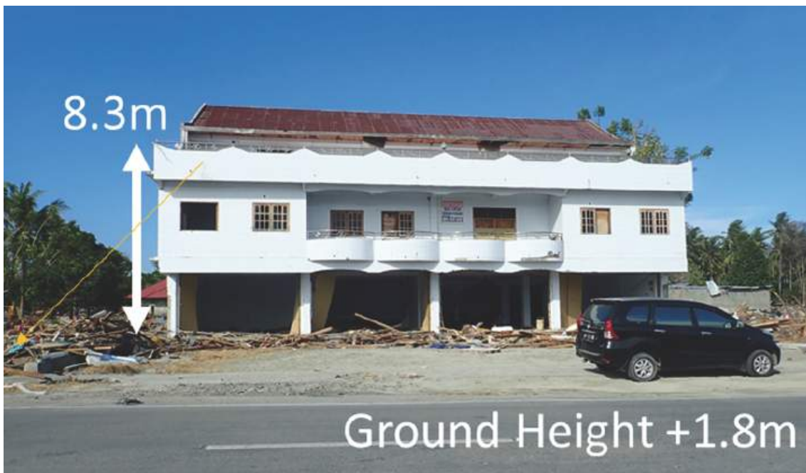
Photo 8 The house located nearby sea, which had some evidence of the splash wave, without tidal correction
