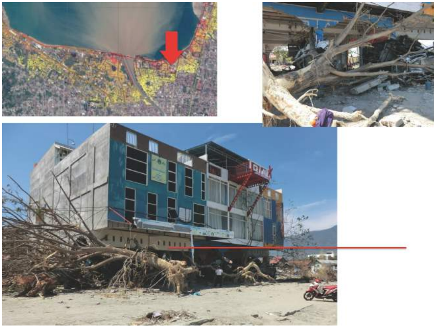
Photo 1 Damaged house where the debris such as trees, cars and motorcycles affected the 1 st floor
