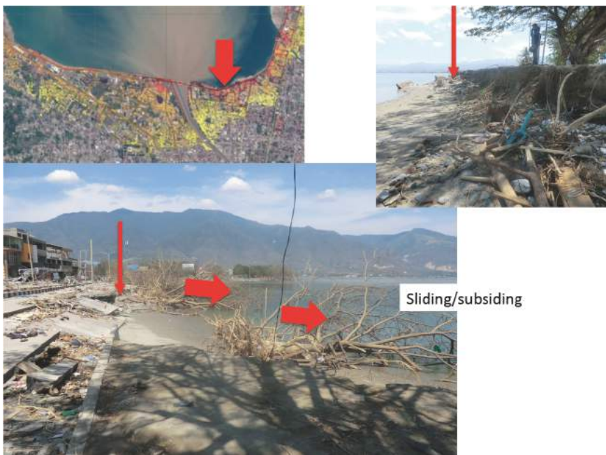
Photo 2 damaged coastal area where the subsidence in large area and backward trees to the sea are observed.
