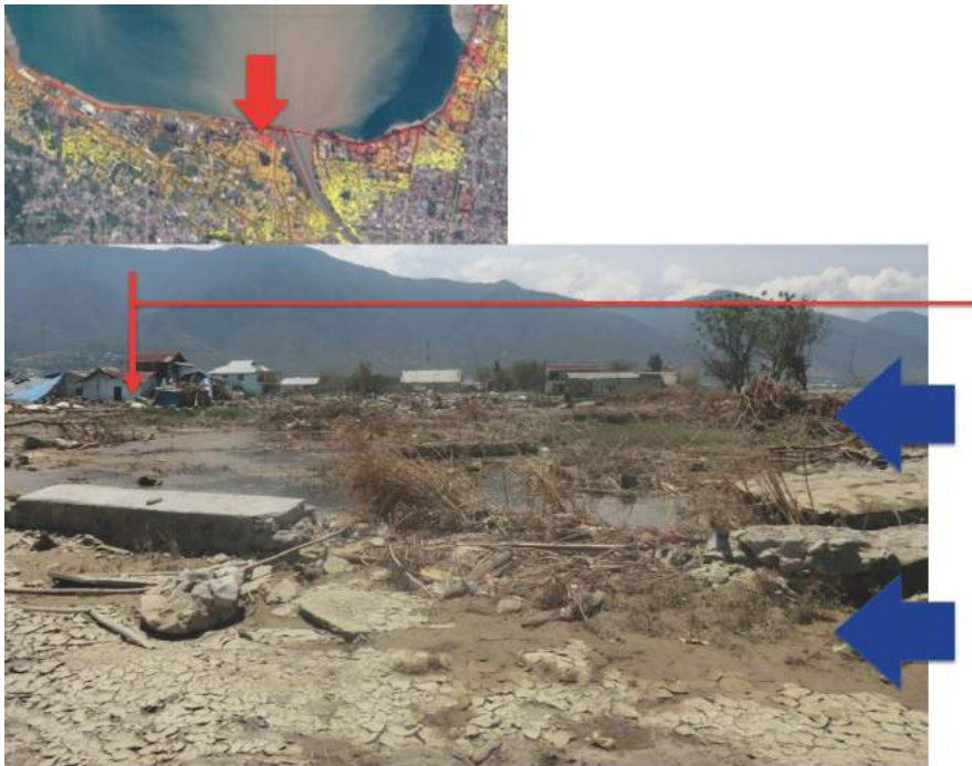
Photo 3 Damaged area due to the strong current of tsunami, causing scouring or erosion on the land where no houses remains.
