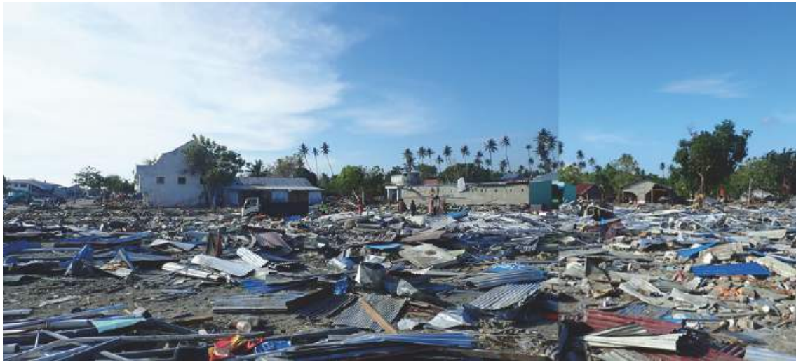
Photo 7 The destruction status at Mamboro
