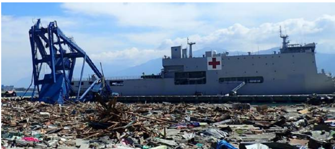
Photo 6 The gantry crane was inclined and almost fallen at Pantoloan
