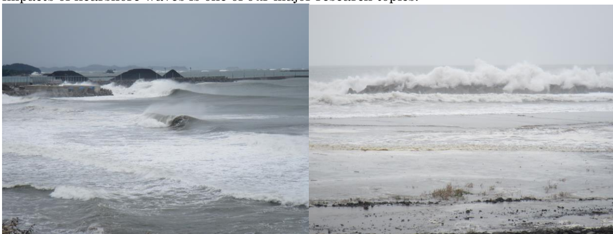
(Left) Wave overtopping of the breakwater near Sendai Shinko. (Right) Wave overtopping of tetrapod-based breakwater near Arahama Beach. Local wave runup up to the gravel road on the beach is visible in the lower part of the picture.
