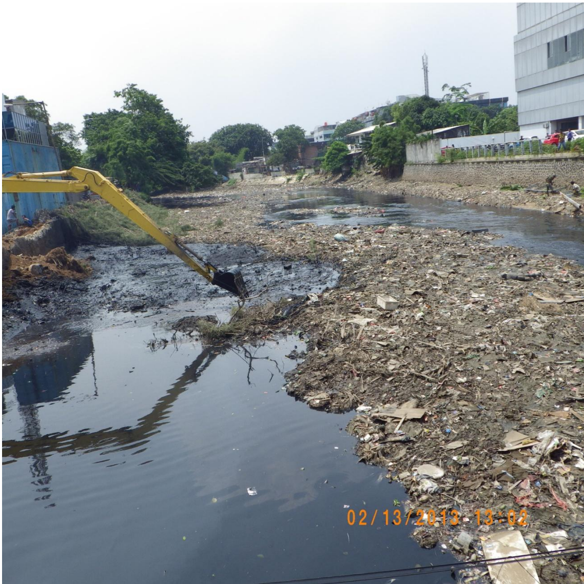
Figure 4.6.2. Sedimentation and trash in the canal leading into Pluit sump.
