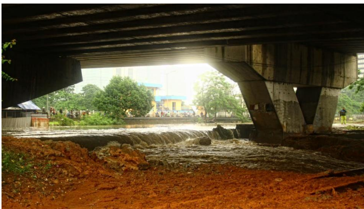
Figure 4.4.10. Photo by Hengki Eko Putra during canal failure. Note the bridge pier on the embankment at the downstream end (right-hand side) of the breach.
