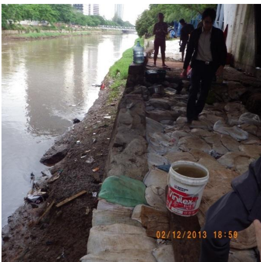
Figure 4.4.7. Downstream end of breach site, looking downstream (west). Note the remains of masonry atop the concrete wall between the sandbags and the parapet wall downstream. Note also that the parapet wall rises in elevation downstream of the breach site.
