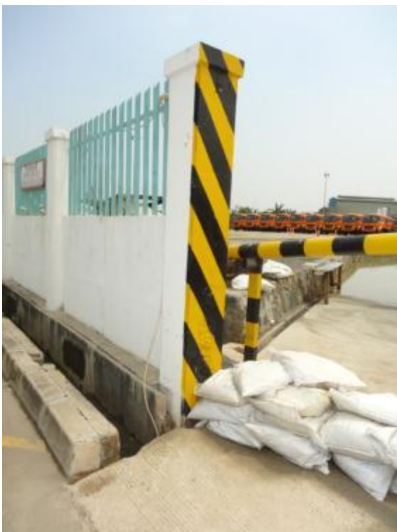
Figure 7.3.3. Strong reinforced concrete wall as countermeasure against flood.
