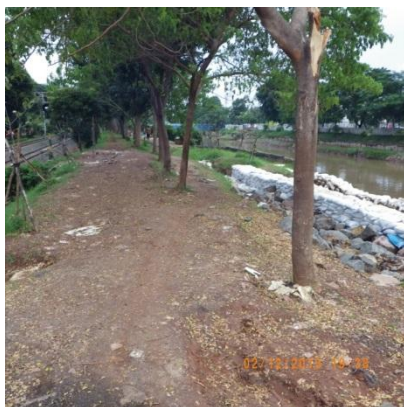
Figure 4.4.4. Trees on the canal embankment crest at the upstream end of the breach location.
