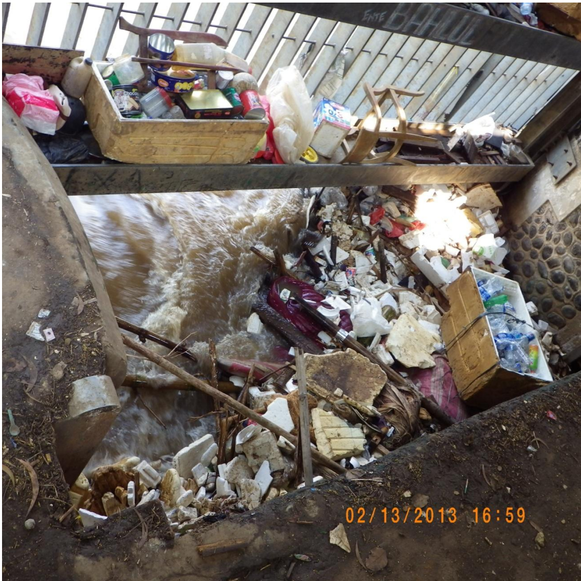
Figure 4.5.2. Floating trash accumulating at the Mangalai (west drainage canal) gate, where flow dives into the gate opening.
