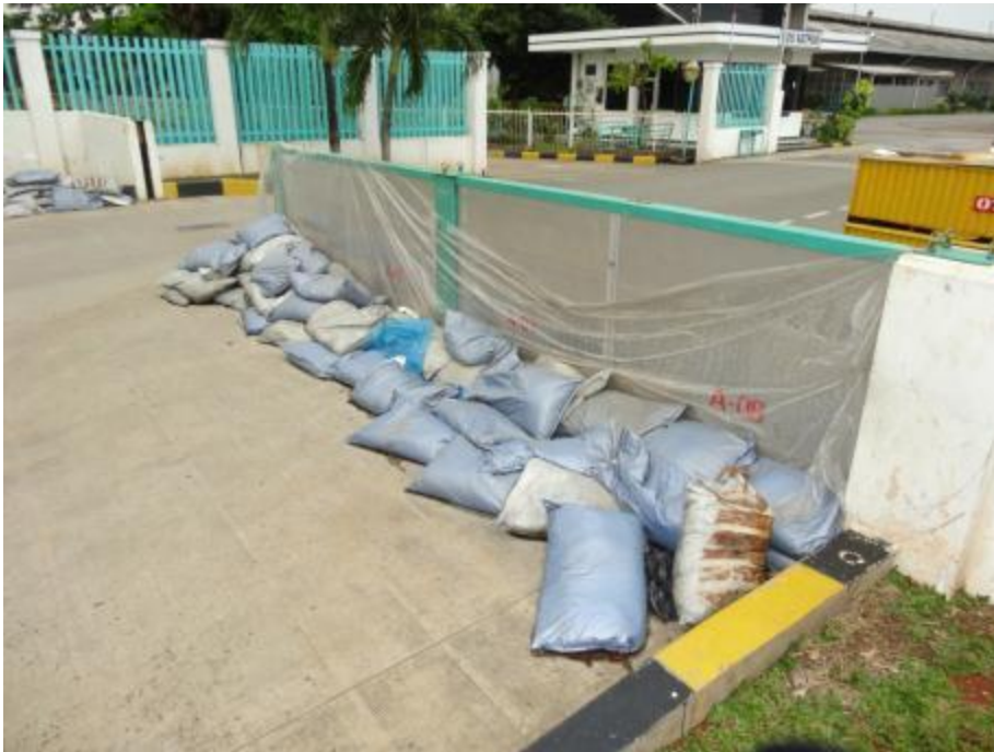
Figure 7.3.6. Sandbags and floodwall.
