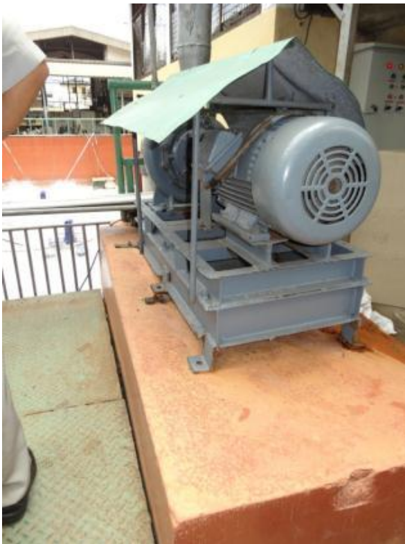
Figure 7.3.5. Elevated fixed drainage pump at private company site.
