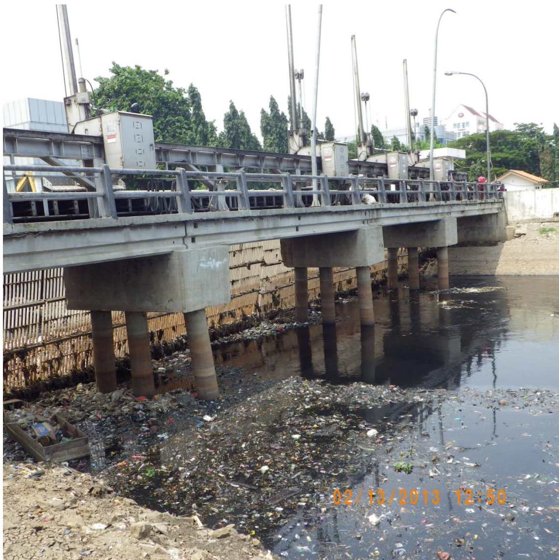
Figure 4.5.3. Trash screens at the entrance to Pluit sump. Were these screens raised during the January 2013 flood, to prevent backwater due to debris damming of the screens? Is this SOP?
