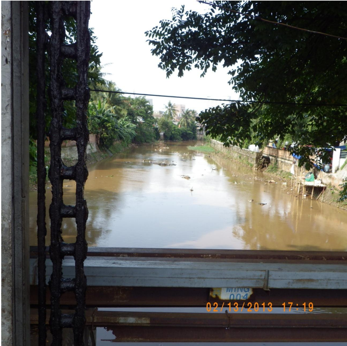
Figure 4.6.3. Sedimentation and trash “islands” in the Old Ciliwung River just below the closed diversion gate. The presence of so much trash just downstream of the closed gate indicates that the gate may have been either opened or overtopped recently.
