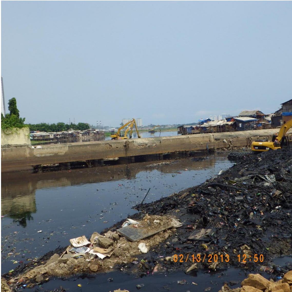
Figure 4.6.1. Dredges operating at the entrance to and inside Pluit sump.
