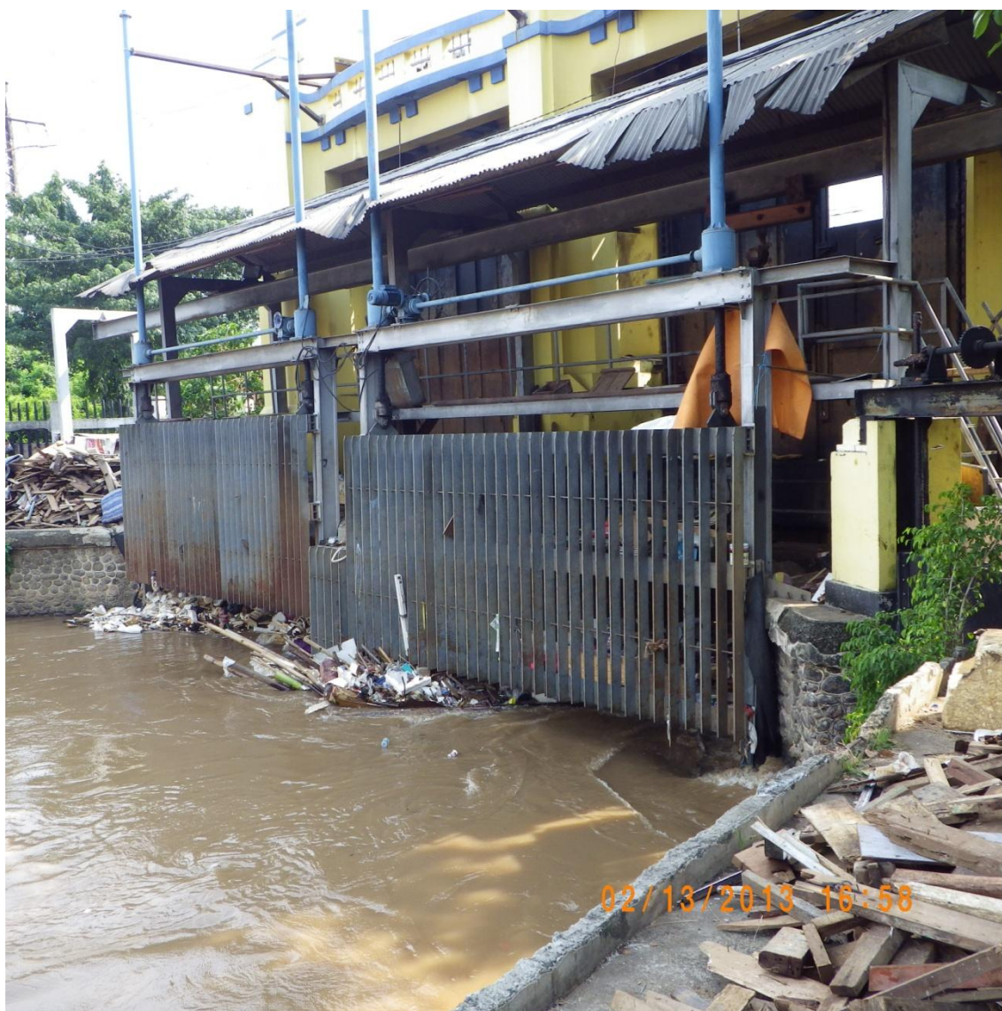
Figure 4.5.1. Floating trash at the entrance to the Mangalai (west drainage canal) lift gates. These gates are always open, as the west drainage canal is the main pathway for water from the upper Ciliwung River to reach the ocean.
