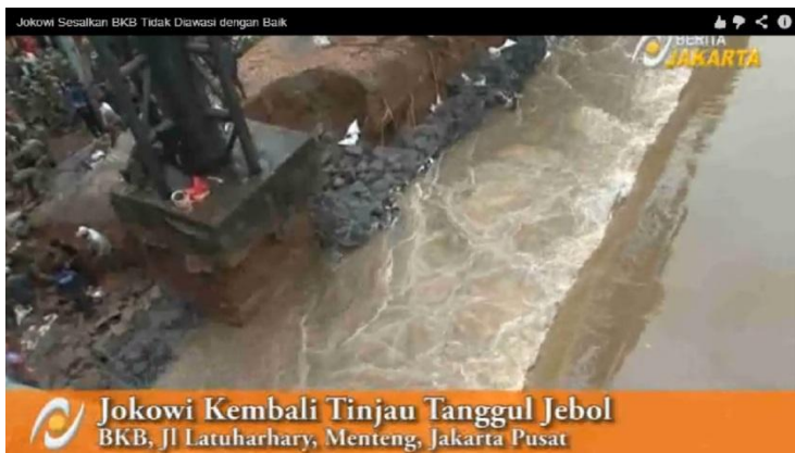
Figure 4.4.5. Video capture image from Jakarta News, showing overtopping of the concrete wall (at water level 3), tree roots in the canal embankment crest, and a tower foundation encroaching on the embankment.
