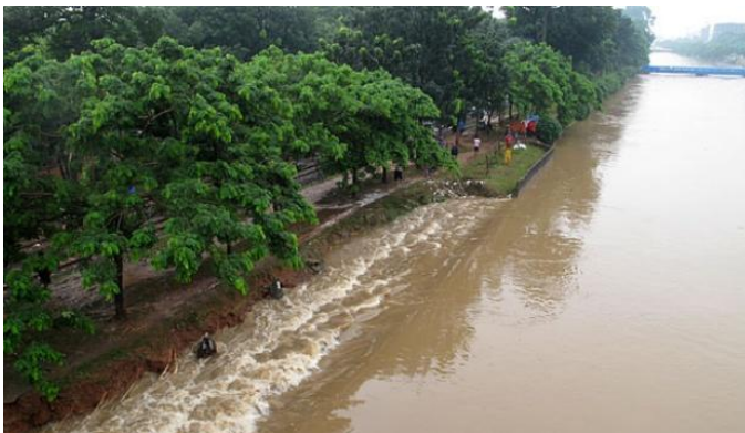
Figure 4.4.6. Photo looking upstream by Hengki Eko Putra during canal failure. Note that the parapet wall on the upstream end of the breach drops in elevation through the breach site.
