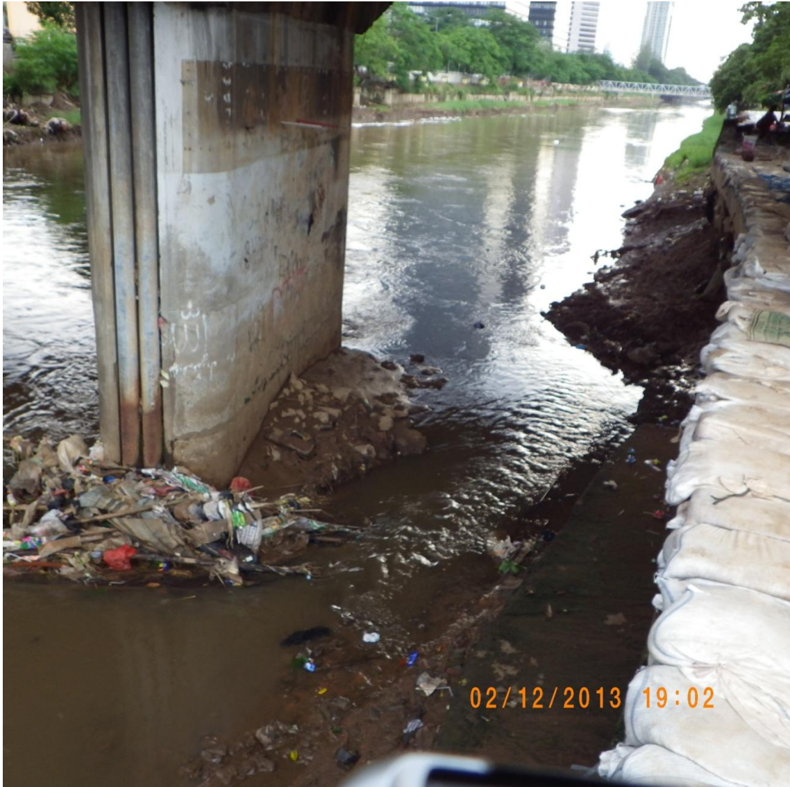
Figure 4.5.4. Trash causing debris damming of the bridge pier beside the site of the west drainage canal embankment breach.
