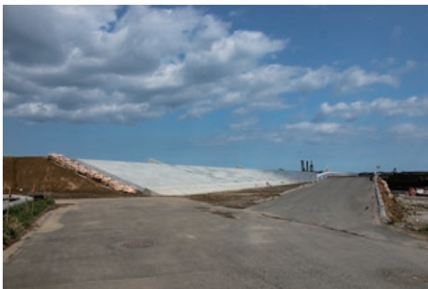
Fig. 4.19 Seawall Under Construction in Natori City
