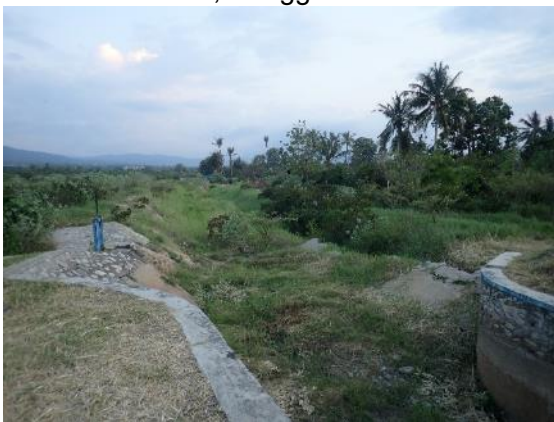
Irrigation may have triggered liquefaction, Jono Oge
