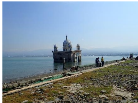
A mosque affected by landslides and tsunamis, Palu Bay
