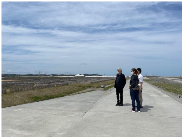
Observing sea wall in Futaba area
