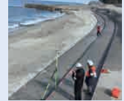
Tsunami trace survey (Kurobe city, Toyama Prefecture)
