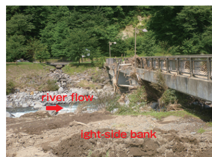
▲ (Photo 3) The Ryu River (Shizukuishi, Iwate Prefecture), normally known for mountain stream fishing. Trees and driftwood caught on bridge girders illustrate the intensity of the flood.
