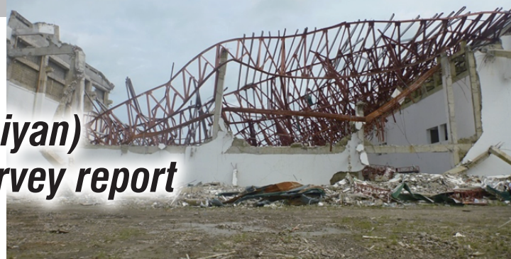
(Photo 1) Leyte Convention Center – an evacuation facility where strong winds caused the roof to collapse.
