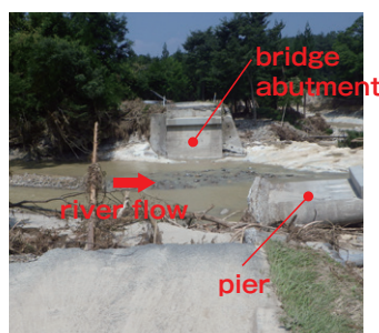
► (Photo 2) Collapsed pier at Yabitsu Bridge (Shizukuishi, Iwate Prefecture). Analysis after the survey indicated a river flow speed of over 5m/s at the time of collapse.
