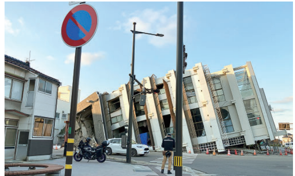
A collapsed office building, Wajima. October 26, 2024.
