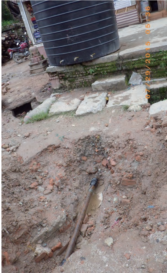
Fig. 5.1.15. Sankhu town. Leaking water supply pipe taped up with pipe wrap.
