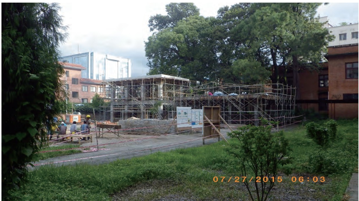
Fig. 5.1.7. JICA demonstration project at Tribhuvan University, Institute of Engineering, showing RC frame construction with brick shear walls. Posters explain the construction techniques.
