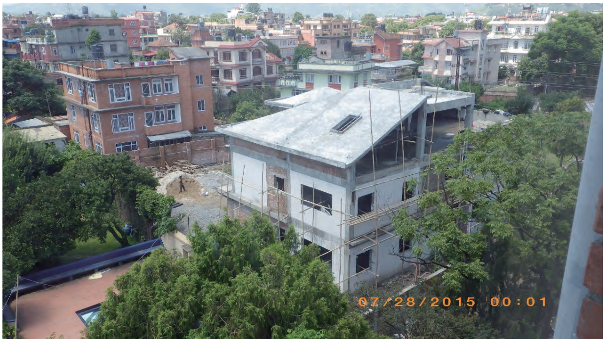
Fig. 5.1.3. House with RC frame and brick shear walls under construction next to Patan Hospital.
