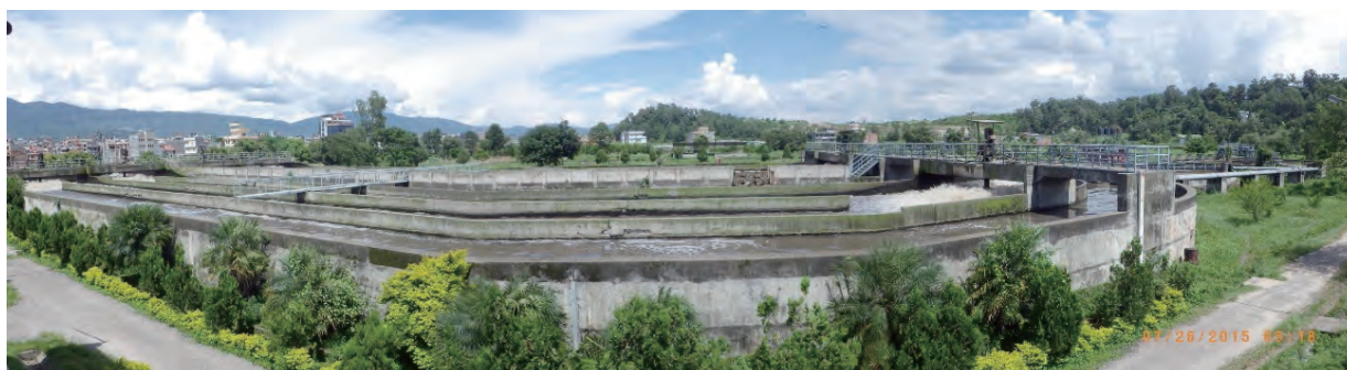
Fig. 5.1.17. Panorama view of Guheshwori Wastewater Treatment Plant. From right to left: primary clarifier, secondary clarifier, aeration flume for activated sludge.
