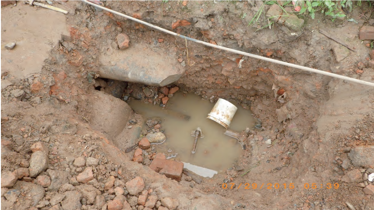
Fig. 5.1.16. Sankhu town. Ruptured water supply pipe beside wastewater pipe or septic tank
