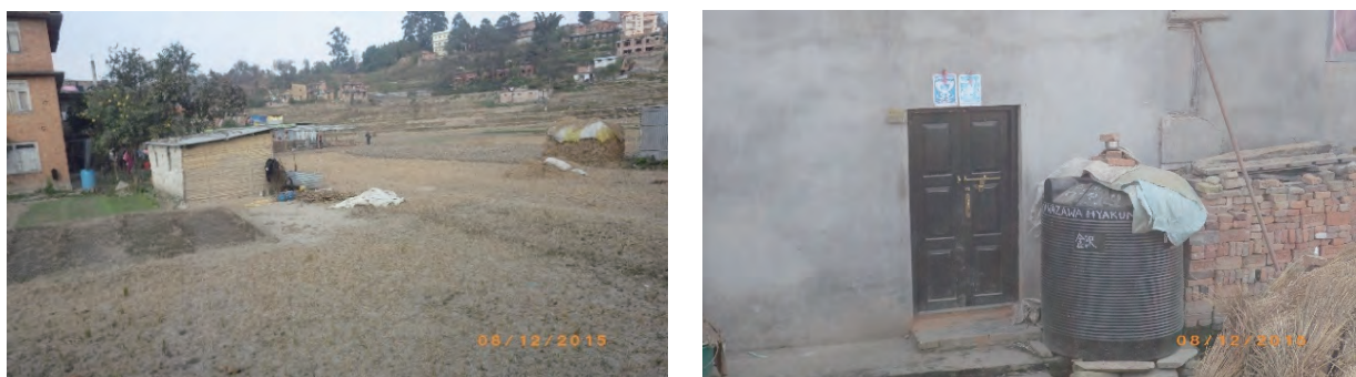
Fig. 5.3.8. The shelter built with combination of bamboo wall and zinc roof in Khokana area (left) and typical water tank and donor's name can be found on the surface of the tank (right).
