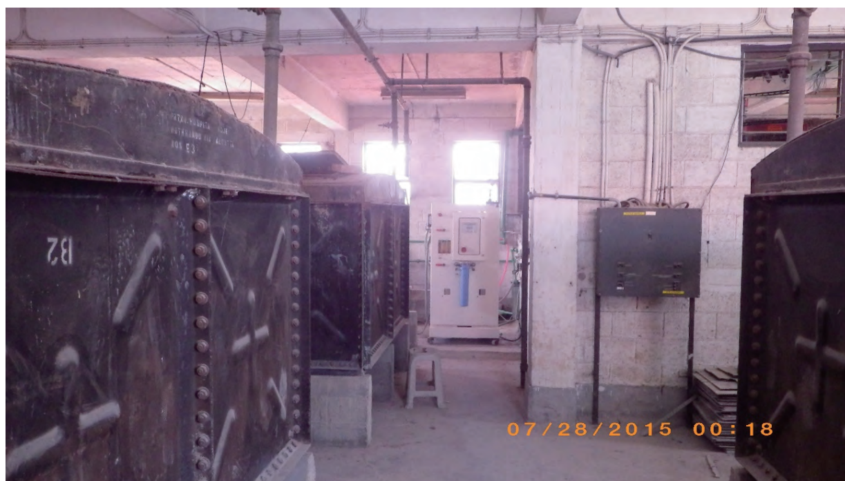
Fig. 5.1.11. Water filter and water tanks on the top level of Patan Hospital. Patan Hospital uses an on-site well for drinking water. Treated chemically. Government water also is treated on site. Two different water systems: drinking water and grey water. Engineers monitor water quality.
