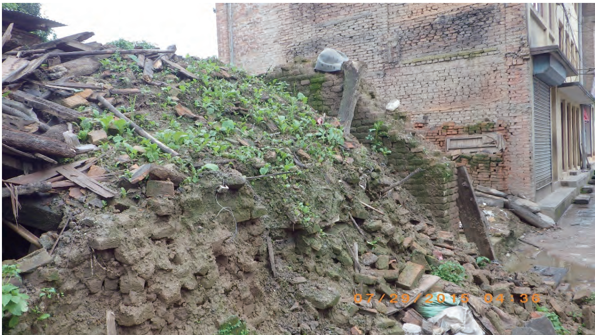
Fig. 5.1.1. Sankhu town. Older homes were built of both fired bricks and adobe bricks. Adobe was the most poorly performing building material during the quakes.
