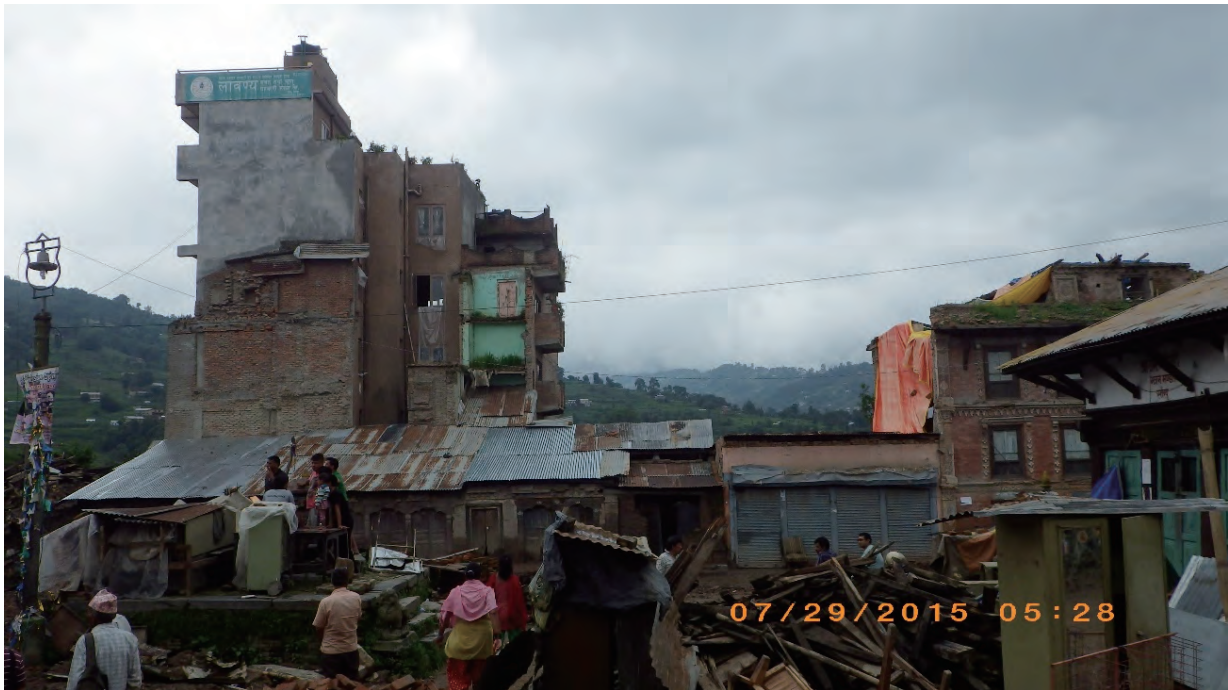
Fig. 5.1.5. Sankhu town. An RC frame building with brick shear walls in the background. In the foreground, an all-brick building had been attached to the RC building's face, but the all-brick building collapsed in the quake. There were many examples of this situation in Sankhu.
