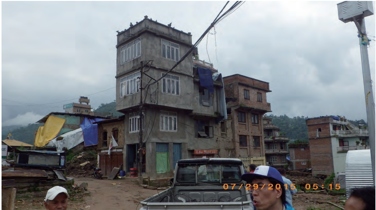
Fig. 5.1.6. Sankhu town. Example of typical soft story and asymmetric construction.
