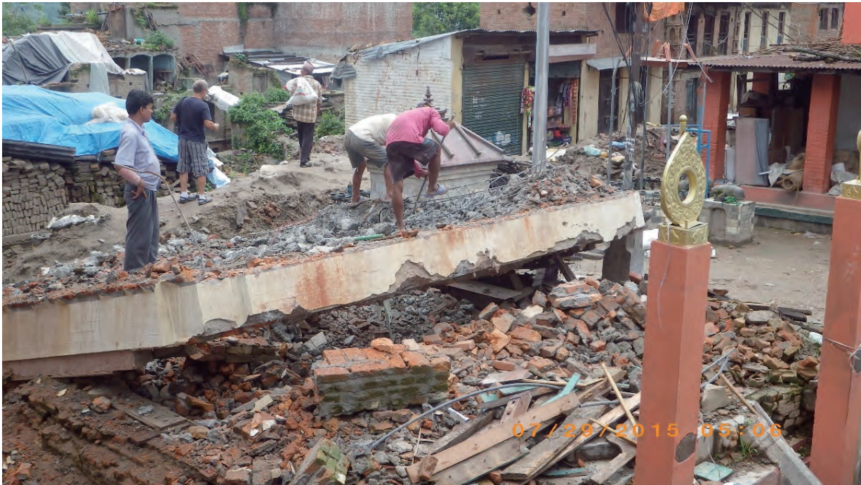
Fig. 5.1.10. Sankhu town. Temple with RC roof slab but brick columns. Columns collapsed.
