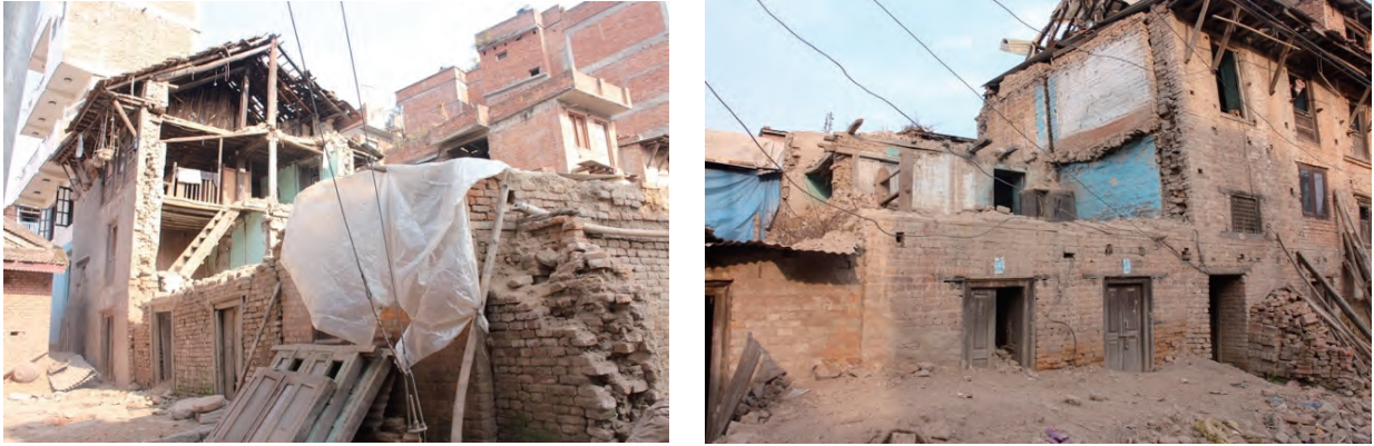
Fig. 5.7.3. a,b, Damaged houses, Khokana, Dec. 2015.
