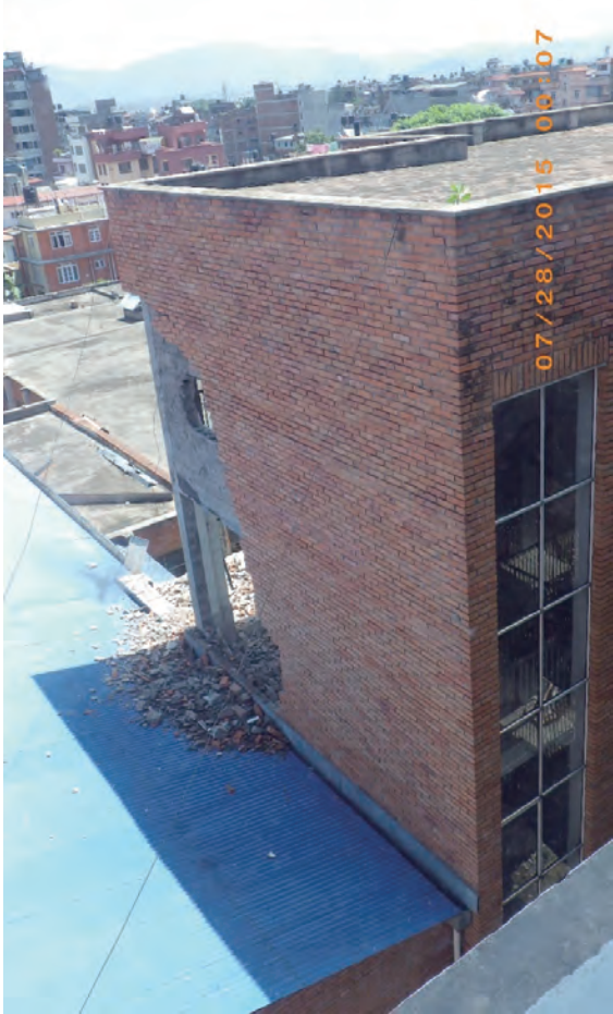
Fig. 5.1.8. Patan hospital old building with damage to brick walls. Concrete masonry frame intact. This building will be repaired and retrofit. The new RC frame hospital building next door was not damaged.
