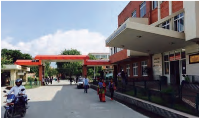
Fig. 5.6.6.b, the Yellow Area was located on the right-side area.
