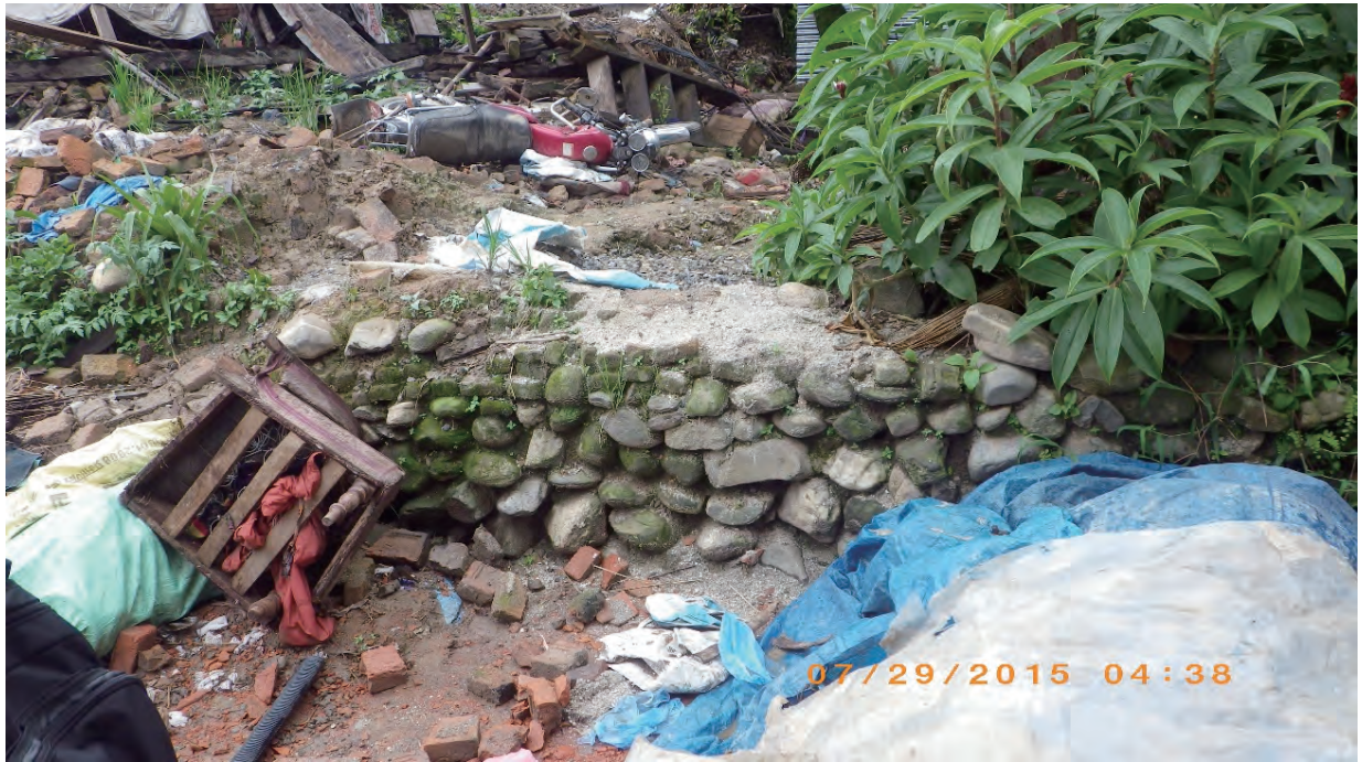
Fig. 5.1.2. Sankhu town. Random rubble masonry was also present, and very weak.
