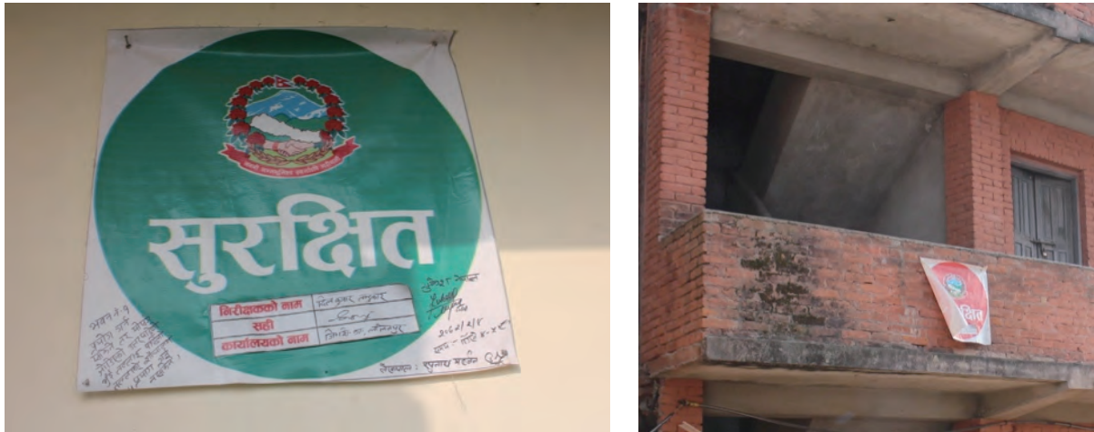
Fig. 5.7.6. Signs showing building inspection results: Left-Green for safe; Right-Red for unsafe.
