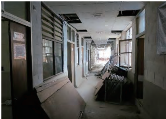
Fig. 5.4.8.c Partially destroyed ward in Patan Hospital
