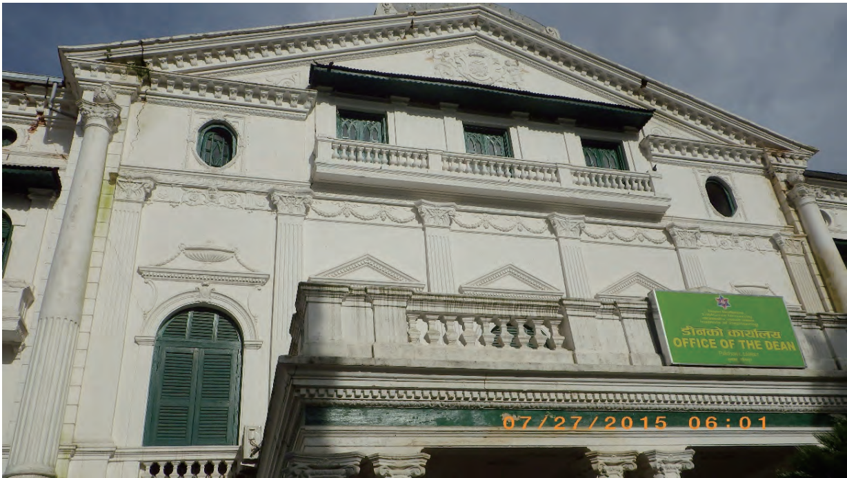
Fig. 5.1.9. Historic brick masonry building at Tribhuvan University, Pulchowk Campus. Damaged by quake and now closed, but faculty are searching for an affordable way to repair and retrofit.
