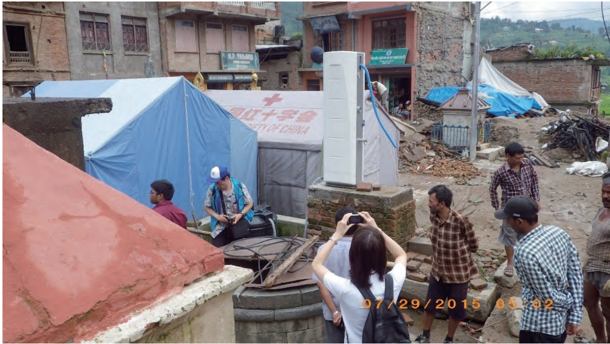
Fig. 5.1.14. Sankhu town. Filter installed by NGO beside well.
