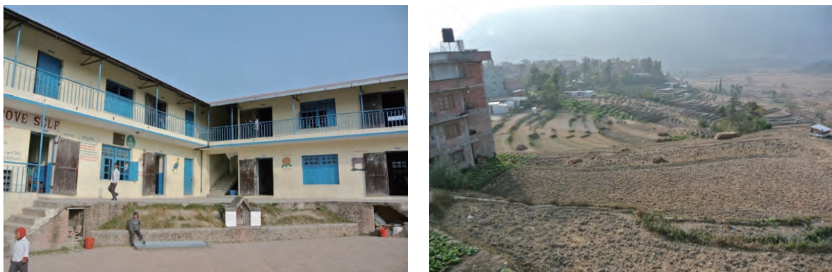
Fig. 5.7.7.a, b. Shree Yuwa Vidhayanth Mandingo Secondary School. Left: School buildings with green signs (safe); Right: view from the School
