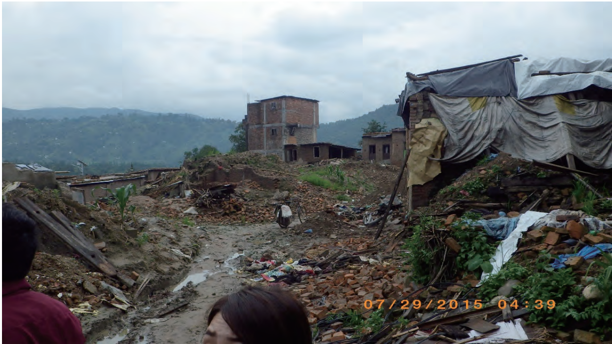
Fig. 5.1.4. Sankhu town. In general, homes of all-brick construction collapsed, but most buildings of RC frame with brick shear wall construction survived.
