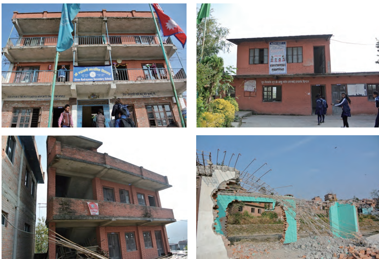
Fig. 5.7.9. Rudrayanee Secondary School. Top left: Main school building (#1); top right: building that survived (#3); lower left: damaged unsafe school building, red sign (#6); lower right: remains of a school building after demolition (#7)
