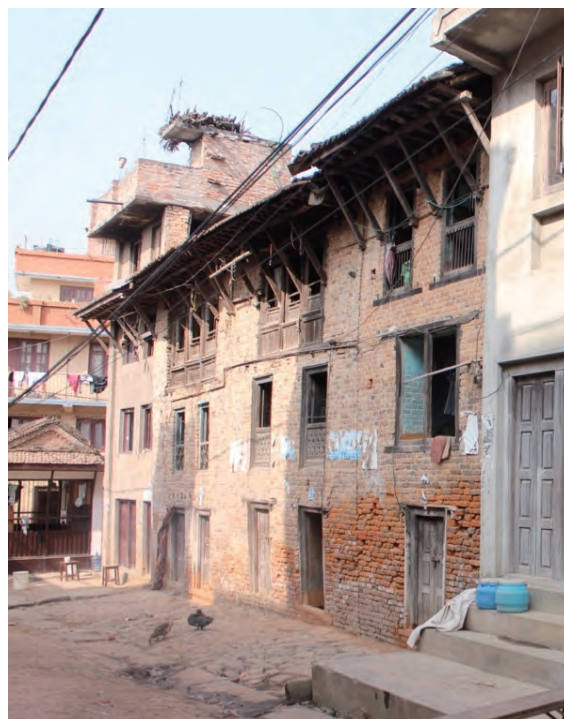
Fig. 5.7.2. Traditional building in Khokana
