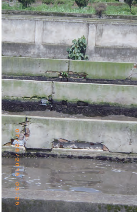
Fig. 5.1.18. Guheshwori Wastewater Treatment Plant. Earthquake damage to partition walls in the aerated activated sludge flume.
