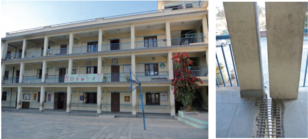
Fig. 5.7.10. Adarsha Shilayubak Secondary School. Left: Attached school buildings; right: gap between of the building blocks, 2 nd floor
