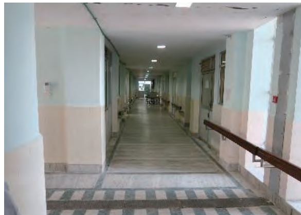
Fig. 5.4.8.d Retrofitted ward was fully functional
