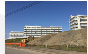
D) Construction of Disaster Public Housings
