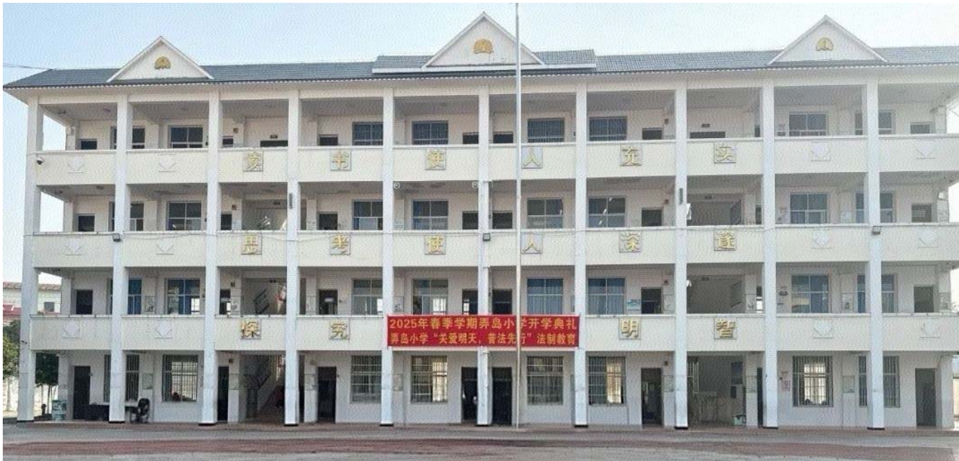
Nongdao Central Primary School RC frame 4-story above ground
