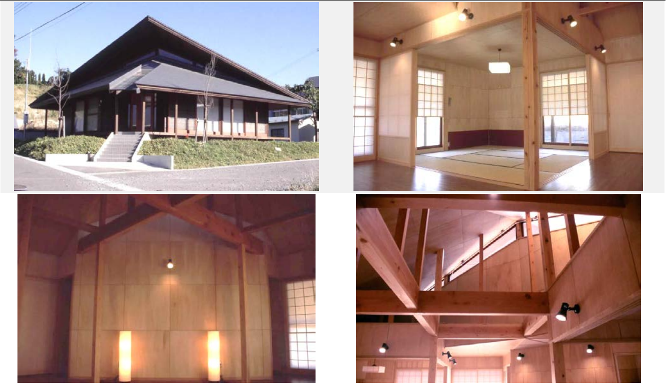
"FUKADAWA Community Hall" with wooden deep eaves MIHARU in Fukushima Pref.
