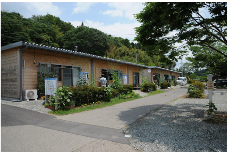
Photo 19-1. Wood-frame temporary housing by the Miharu Reconstruction Housing Association, a group of local construction companies in Miharu, Fukushima Prefecture. It was built on the grounds of the park using the current greenery. These are comfortable temporary houses with the scent of wood, which use a lot of natural wood for both interior and exterior, and at the same time consider high heat insulation and high airtightness. Residents also highly evaluated these temporary houses. (Photo by Iwata)
