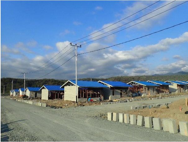
Figure 46-2. Tondo relocation site under construction
