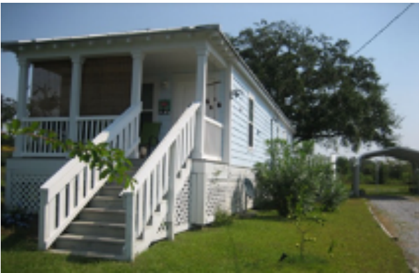
Figure 47-2. Mississippi Cottage converted into permanent housing
