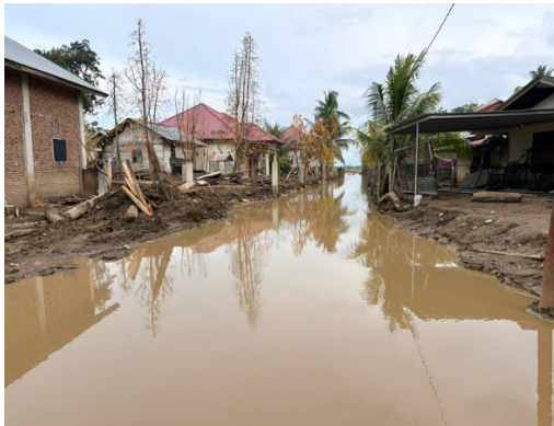
Flooded house in Pidie Jaya 2 months after Senyar, North Aceh
